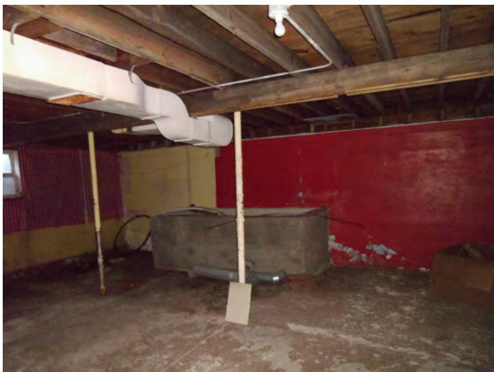
Figure 13—Church basement with baptistry (author's image)
