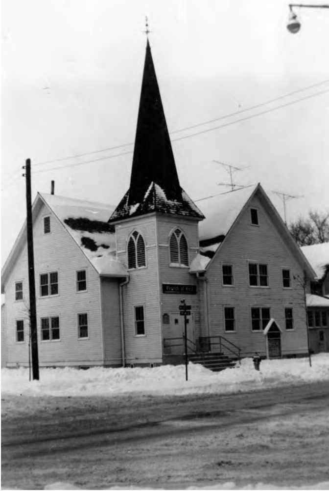
Figure 12: Remodeled Church after fire (courtesy of Wilferd Felchle)
