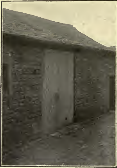
OLD BARN, SILSDEN, WHERE THE FIRST SERVICES WERE HELD.
