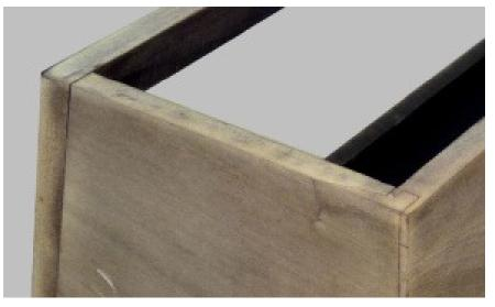
Stripped cabinet showing locking rabbet joints used on back of cabinet and on construction of the battery box.
