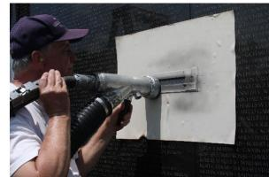
meticulous work to match the stroke and depth of the surrounding names to within 1/1,000 of an inch. The physical work of adding the names and changing designations will be performed by James Lee of the Colorado-based company (Engrave Write).
