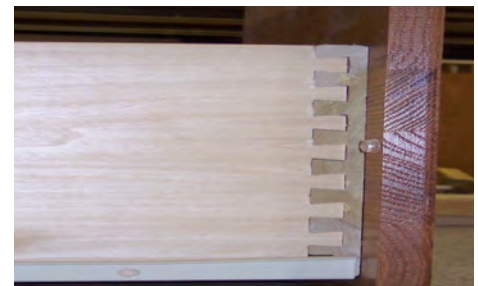
Dovetail Construction
