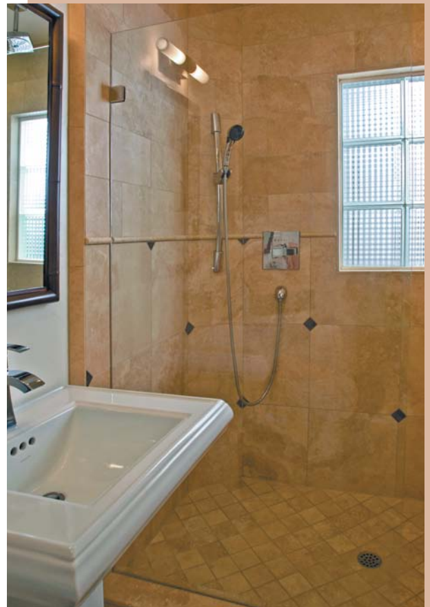
This shower delivers accessible Universal Design. Three showerheads, one an adjustable hand held on a bar, all controlled separately, deliver maximum shower capability. Endless hot water via a tankless water heater was included. Instead of a built in seat, the clients opted for blocking in the walls to easily attach a future seat and grab bars. Designer: Adel Visser, CKD, CBD, CID, All About Kitchens & More! www.allaboutkitchens.us Delta shower fixtures. Photography: Gordon Lazzarone.
