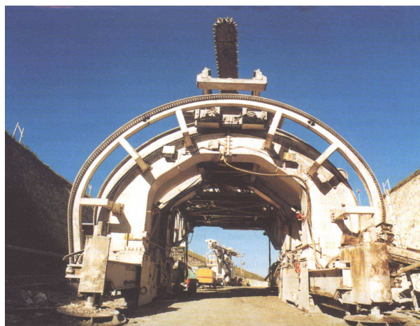
Figure 2. Prevault tunnelling machine.
