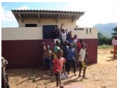
Constructed School Latrine
