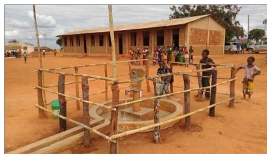
Borehole with hand pump constructed by the Project
