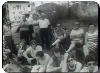
Residents meet to plan their campaign to oppose the Northern Freeway, assisted by the trade union ban on demolition of houses. Photo courtesy of film “The Battle for Bowen Hills” by Peter Gray & Gary Lane.
