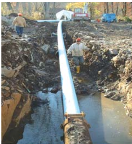
Fig. 2b: Continuous Sliplining
