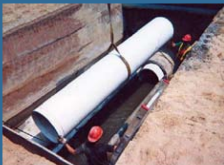
Fig. 2a: Segmented Sliplining
