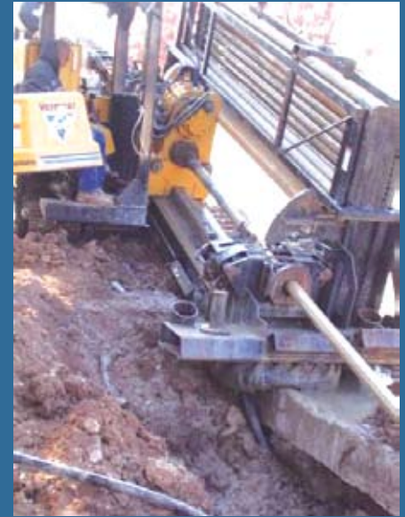
Fig. 1b: Horizontal Directional Drilling (HDD) Method
