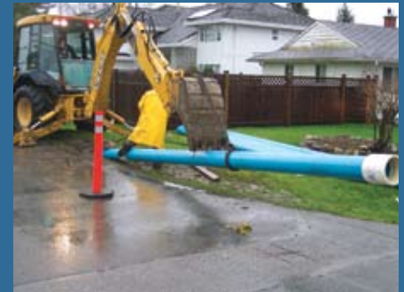
Fig. 1d: Horizontal Directional Drilling (HDD) Method
