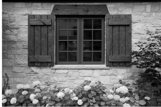
http://www.pickellbuilders.com Photography by Linda Oyama Bryan. Stone and Stucco French Provincial with Hand Hewn Window Headers and Shutters on Lake Geneva.
