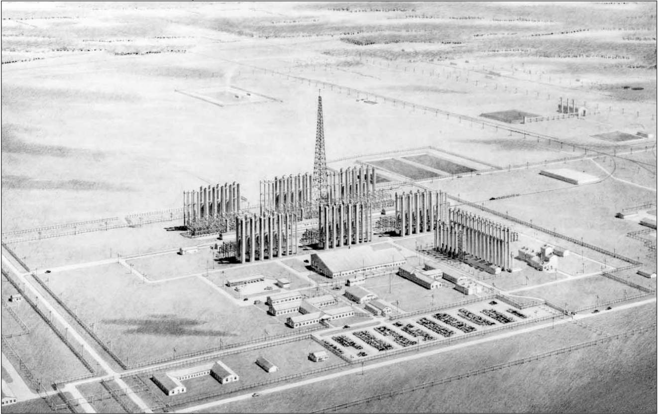
Birds Eye View of Dana Plant, Dana, Indiana. Dana had a more compact layout with the flare tower placed between the GS units. Savannah River, Dana Area, Env. 22. Courtesy of the Hagley Museum and Library.
