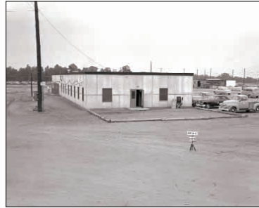
Office and Change House
