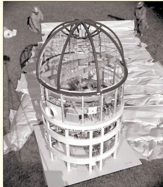
Model of the Heavy Water Components Test Reactor built in Wilmington prior to start of its construction at the site in B Area in 1959. Courtesy of SRS Archives, negative 7081-1.
