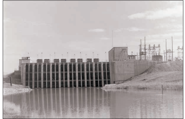
River pumphouse supplied river water to D Area. Courtesy of SRS Archives negative 3178-5.
