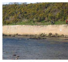
A previously eroding terrace bluff on the outside of a meander bend, stabilised by a concrete revetment to protect a nearby road (© The James Hutton Institute).
