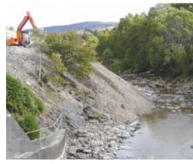
Gravel replenishment on the regulated River Garry, Perthshire. Gravel trapped behind a weir has been excavated and re-deposited below the weir to restore sediment supply to reaches downstream (© Chris Gibbins, Northern Rivers Institute).
