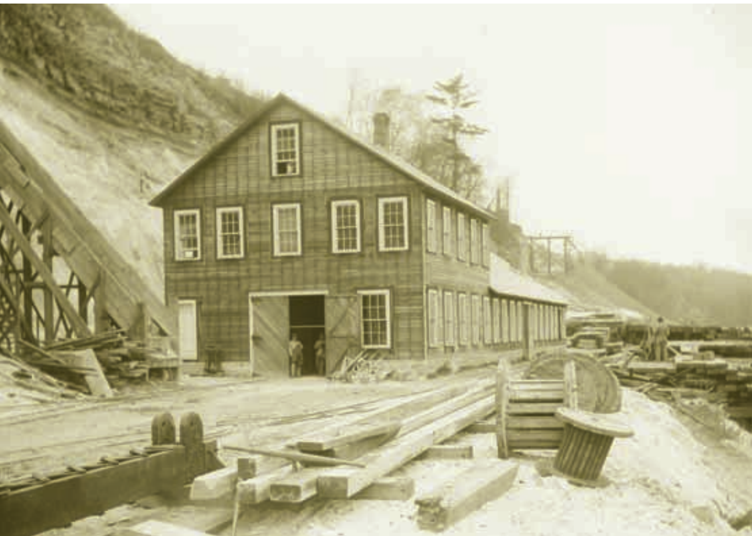
Work site for Lock and Dam No. 1 in 1907, before construction stopped
