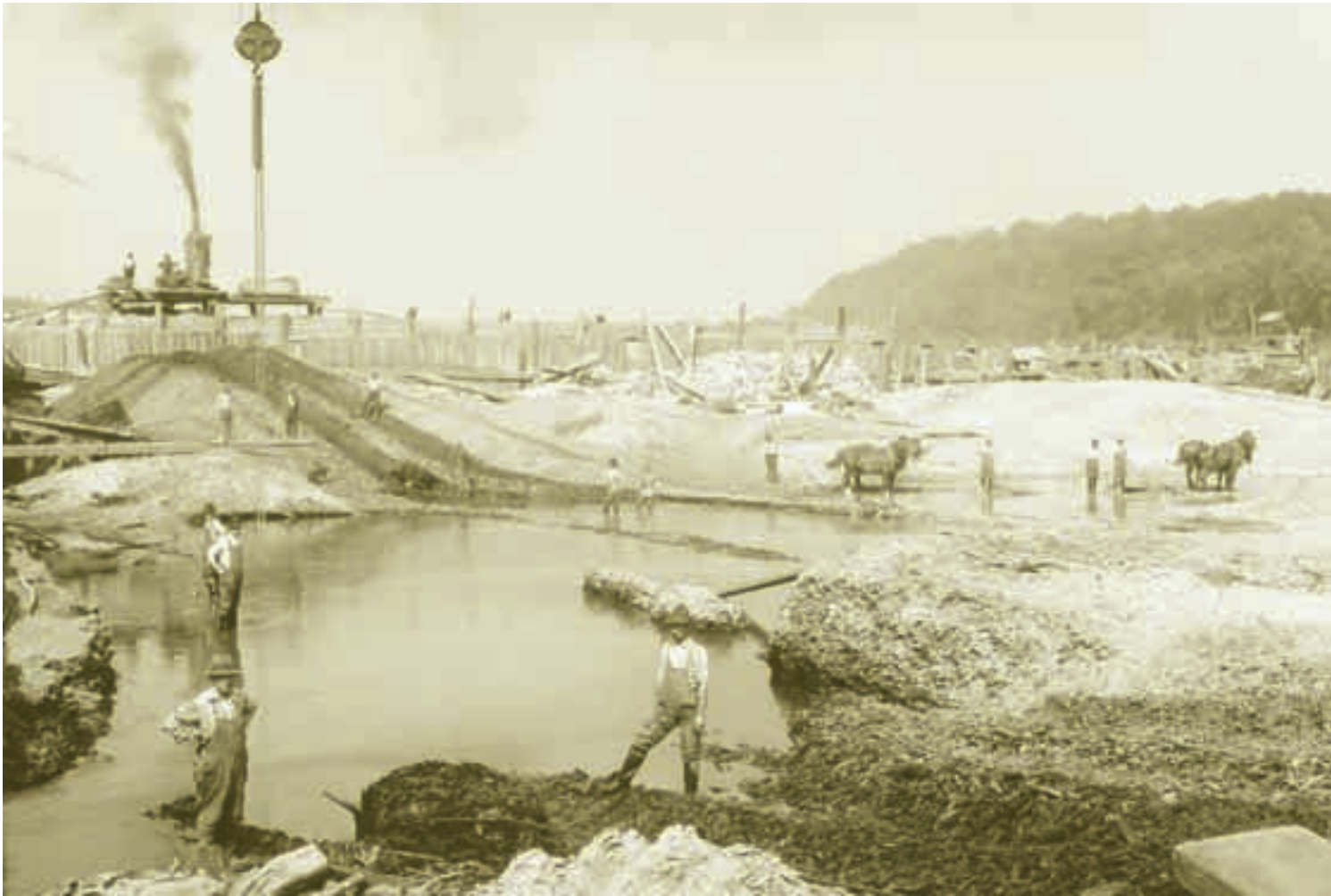
Men and animals laboring to complete Lock and Dam No. 1 in 1914
