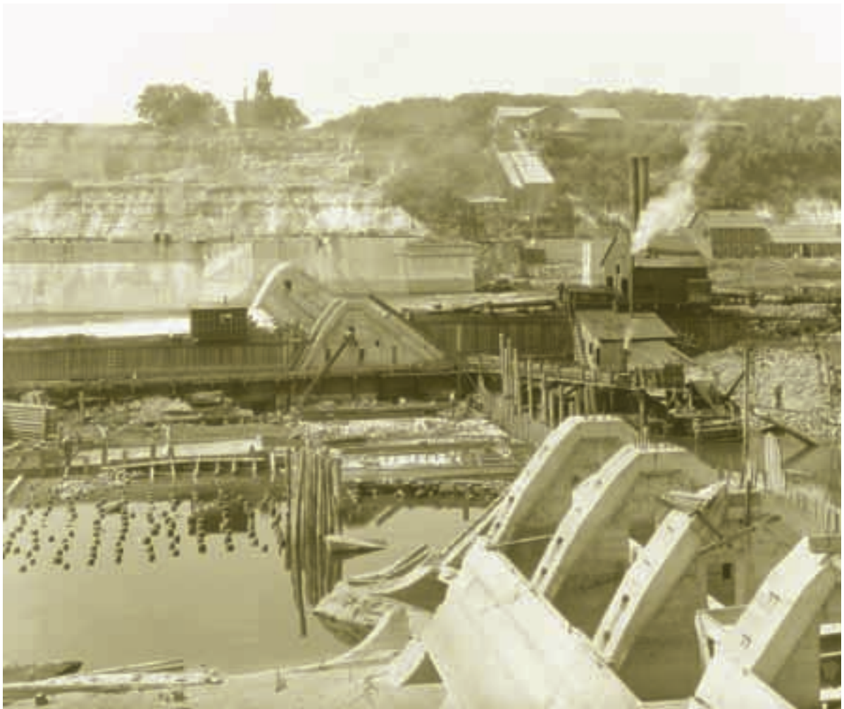
Lock and Dam No. 1, showing innovative prefabricated design that allowed for cold-weather construction, nearing completion, 1916
