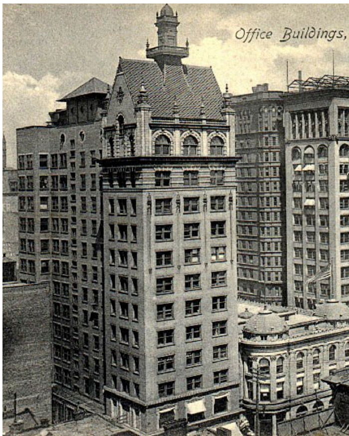
The Holland Building, showing parts of the Chemical Building and the Union Trust Building to the right. From a postcard entitled "Office Buildings, St. Louis, U.S.A." Courtesy of Michael Allen.
