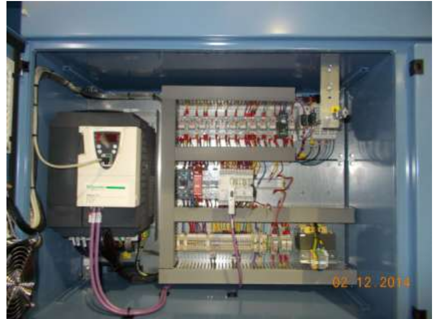
An 11 kW VSD compartment in an IMCC
