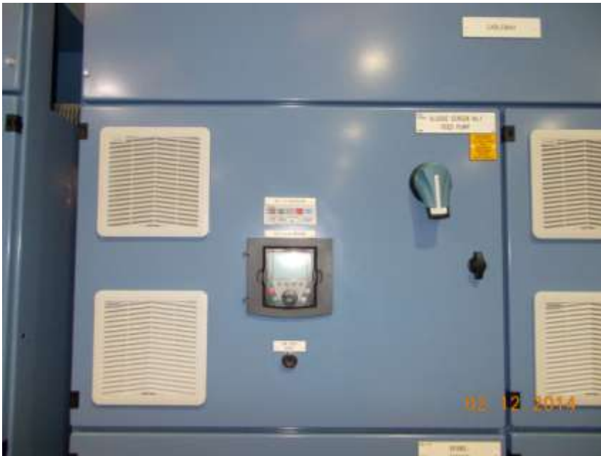
An 11 kW VSD compartment in an IMCC
