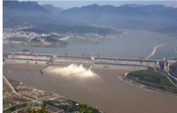
Figure 2: Two deep holes and a trash way hole open for sluicing the mounting flood water at the Three Gorges Dam. Credit: http://english.people.com.cn/90001/90783/91300/6691772.html
