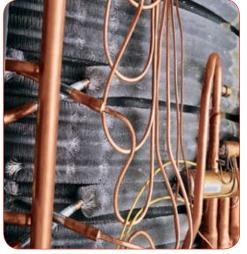
A typical 2-1/2 ton air conditioner or heat pump requires 30 or more brazed joint connections in the coil. A modern Trane unit of the same size requires only 10 with Spine Fin."
