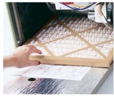
The dual door latch design of our upflow furnaces makes the filter door easy to open so filter changing is a breeze for homeowners. This helps maintain system performance over the long haul.
