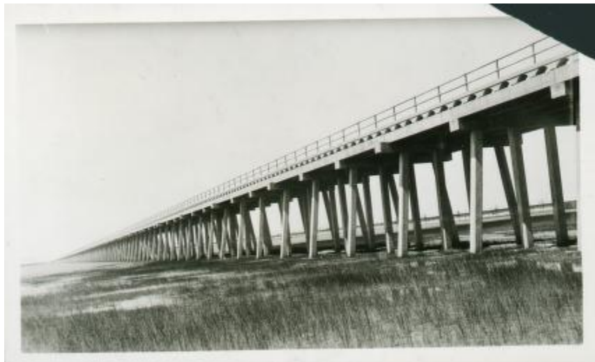
CAUSEWAY--CALIFORNIA STATE HIGHWAY--BETWEEN SACRAMENTO AND DAVIS. CONCRETE CONSTRUCTION. COST $400,000.00. LENGTH 3 1-10 MILES; WIDTH 26 FEET. DEDICATION SACRAMENTO MAY 11TH TO 14TH, 1916.
