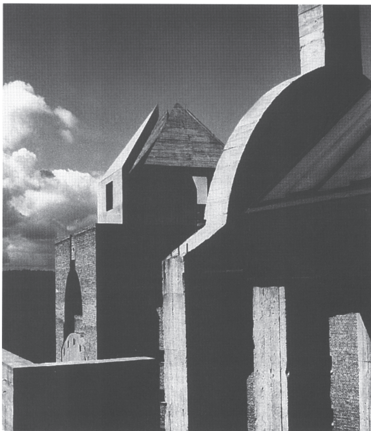
Plate 7 The Way of Four Doors, High Seminary of the Fraternity of the Fathers of the Resurrection, Kraków, Father Pawlicki Street 1983–8 (Dariusz Kozłowski (with colleagues))
