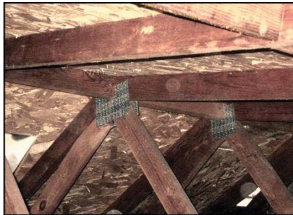
Photo: 9. View of sub-roof. (1)
