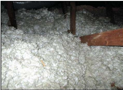
Photo: 9. View of attic insulation. (1)
