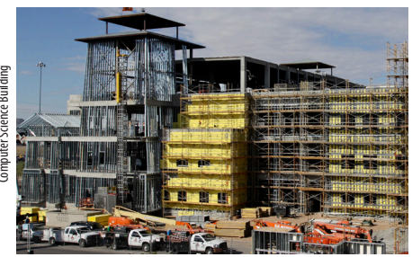
Construction of the new Chemistry and Computer Science Building
