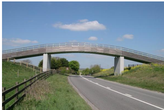
Fig. 3 Itford Farm Bridleway Bridge
