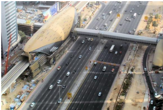
Fig.4 Dubai Metro station and typical access footbridge
