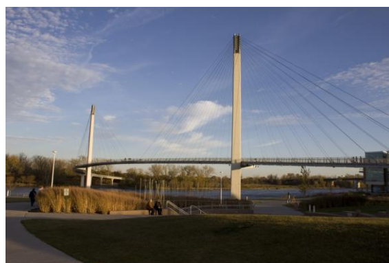
Fig 16 Bob Kerrey Pedestrian Bridge
