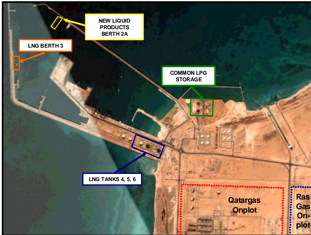
Figure 2: RasGas Expansion (RGX) Facilities within Ras Laffan Industrial City
