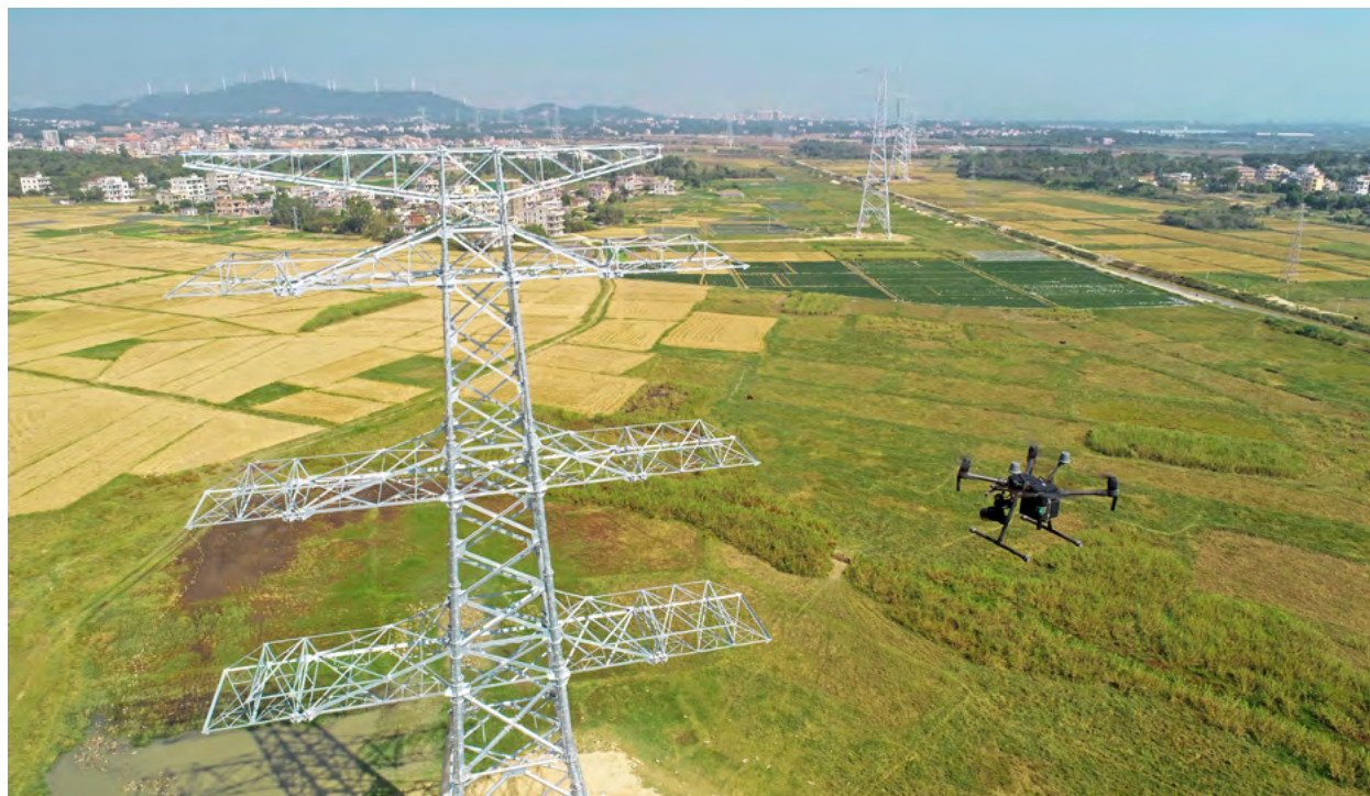
Transmission Tower Inspection. An aerial view of a drone used to inspect a transmission tower (photo by Guangdong Electric Power Design Institute).
