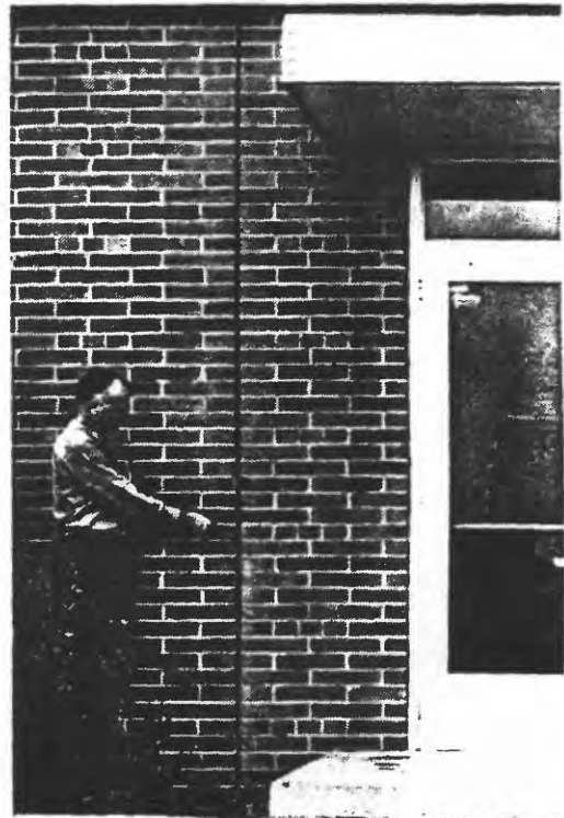
Figure 4. Expansion joints cut into existing walls to allow for future expansion.
