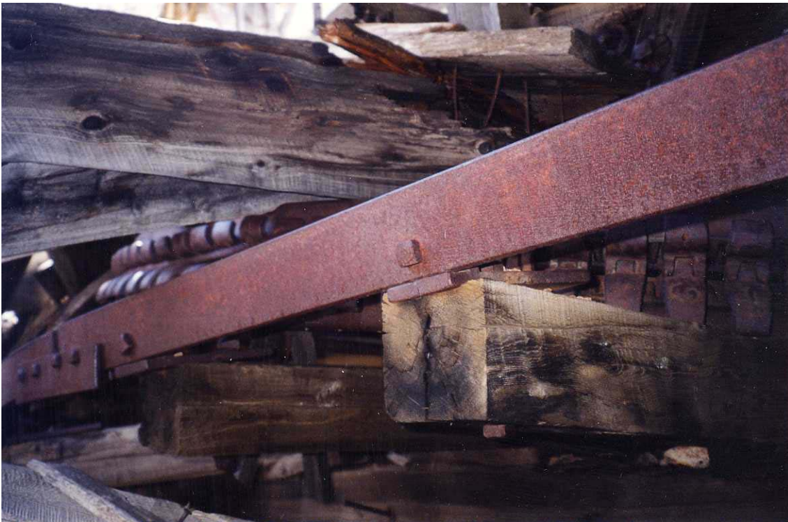
Figure 4-23. Detail of loading rail adjacent to traction rope bull wheel. The cars slid off the track rope onto the rails that led them around the bull wheel and back onto the track rope leading the opposite direction.
