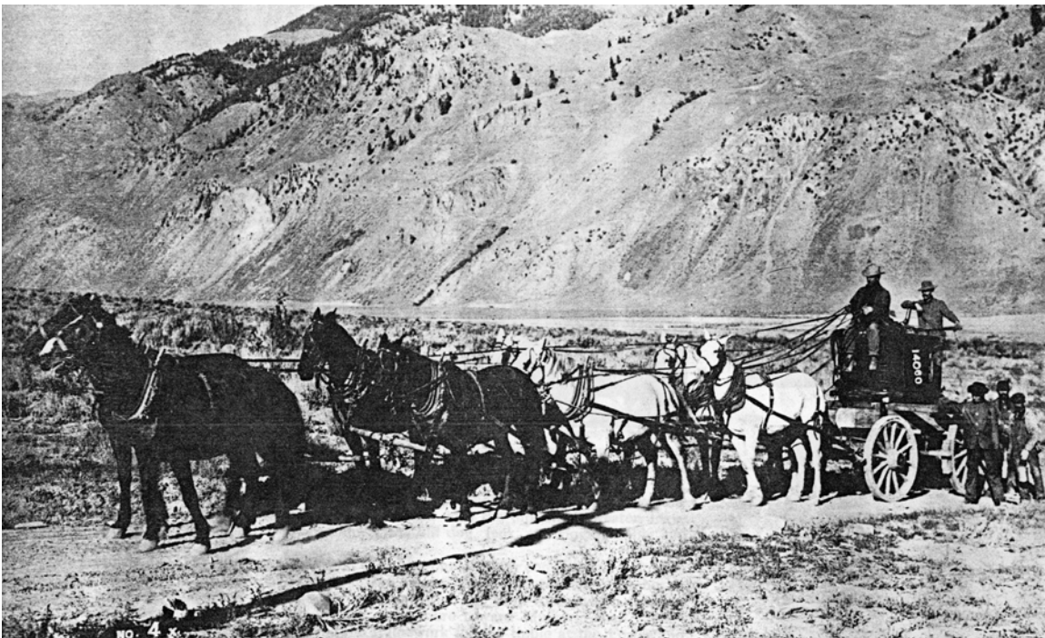
Figure 4-2. Eight-horse team hauling the 14,060-pound tram cable at Aldridge, ca 1906 (Tony Stermitz Photo, from Whithorn and Whithorn 1966).
