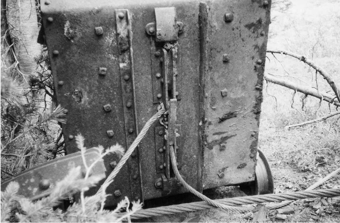
Figure 4-36. Detail of the bottom of a Lawson-style bucket showing how the traction rope is attached to the car (1990 GCM file photo).
