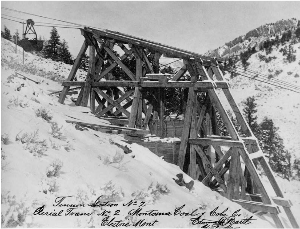
Figure 4-3. Counterweight tower at Aldridge, ca. 1909 (Montana Historical Society Archives).
