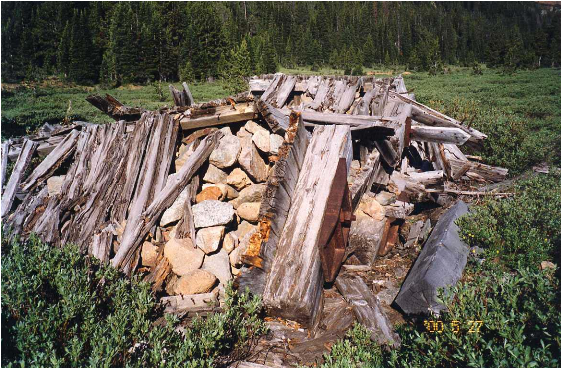
Figure 4-41. The remains of a collapsed counterweight crib at a tension-control tower.
