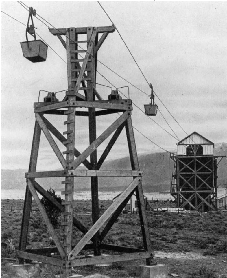
Figure 4-7. A Bliechert-style tram showing support tower and discharge terminal (Trennert 2001).
