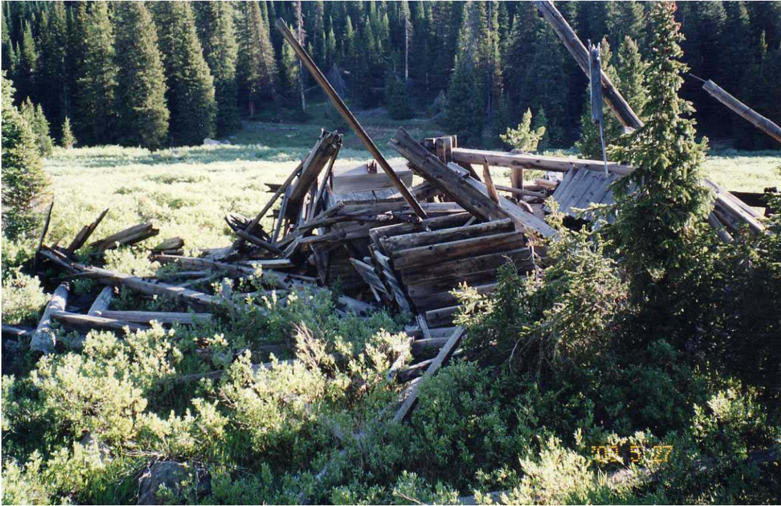
Figure 4-44. Collapsed lower tram counterweight tower remains as they are now found.
