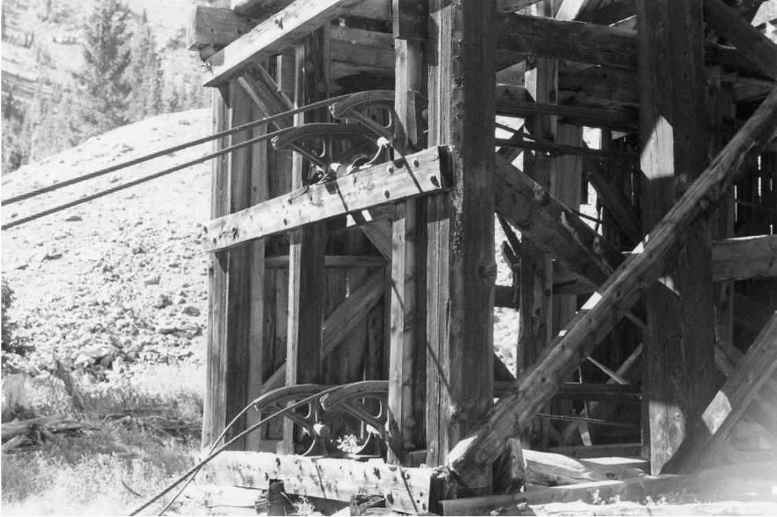
Figure 4-38. The loading terminal of the Lawson-style tram at the Gold Dust ore bin. (1990 GCM file photo).
