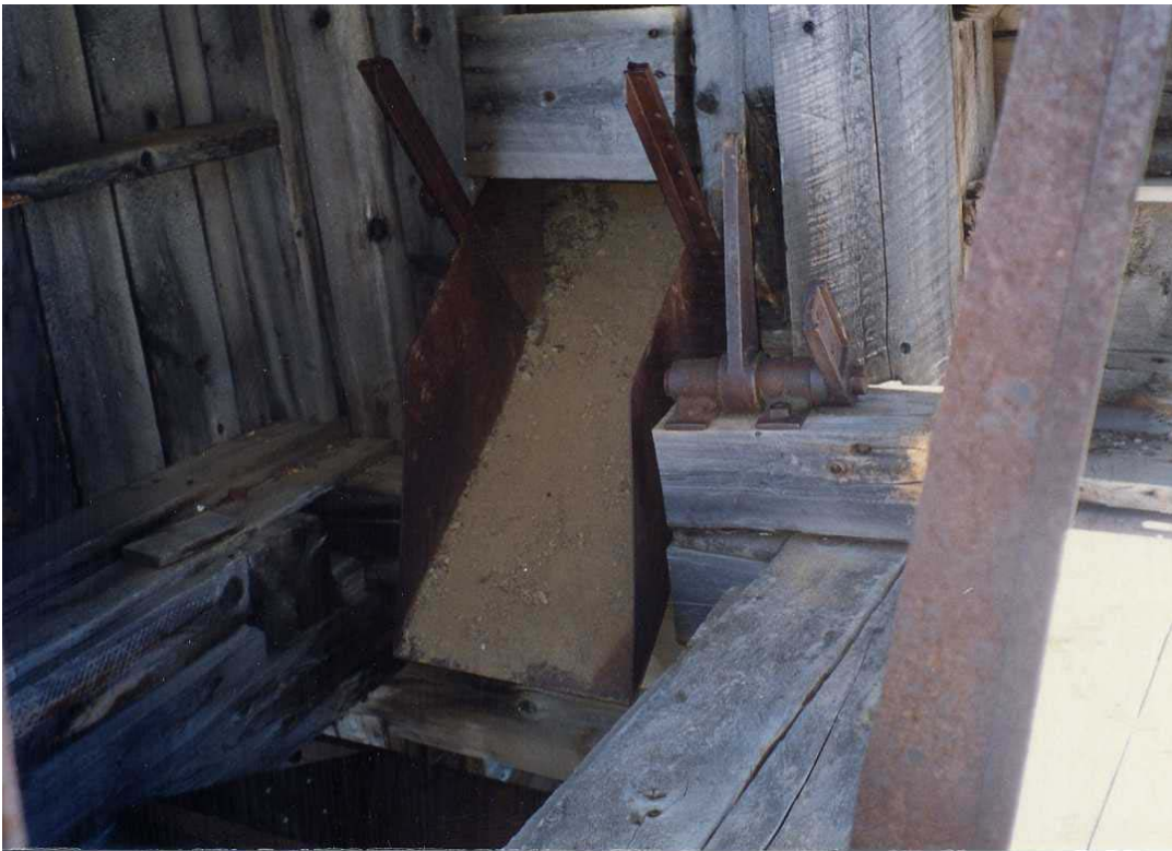
Figure 4-20. Detail of the ore bin hopper at the loading terminal.
