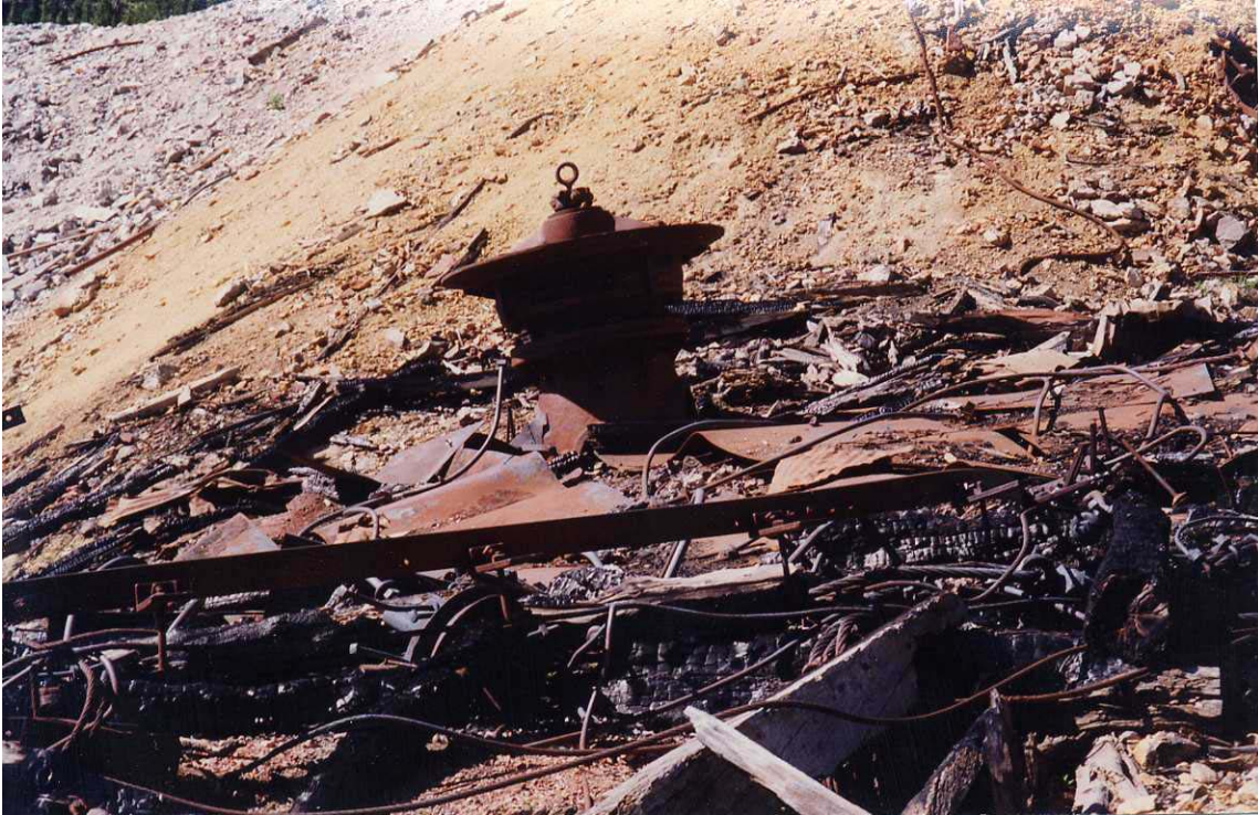
Figure 4-26. The discharge terminal and gyratory crusher (Gold Dust mine Feature 5). Note the cable, sheave wheels and flat iron track. This structure, collapsed as of 1990, was also burned in recent years.
