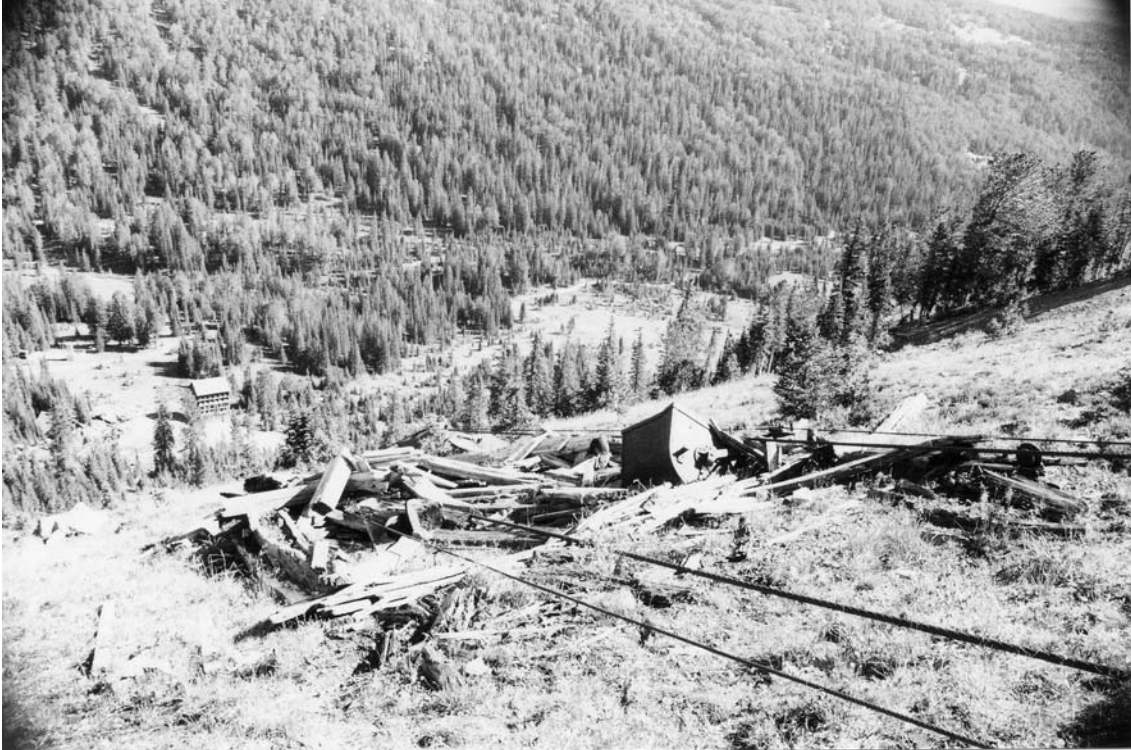
Figure 4-24. 1990 photograph of collapsed support tower. A Bleichert-type ore car can also be seen. Note the large diameter track cable and the small diameter traction rope.
