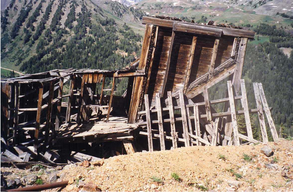
Figure 4-13. The brake house and Homestake ore bin, looking north.
