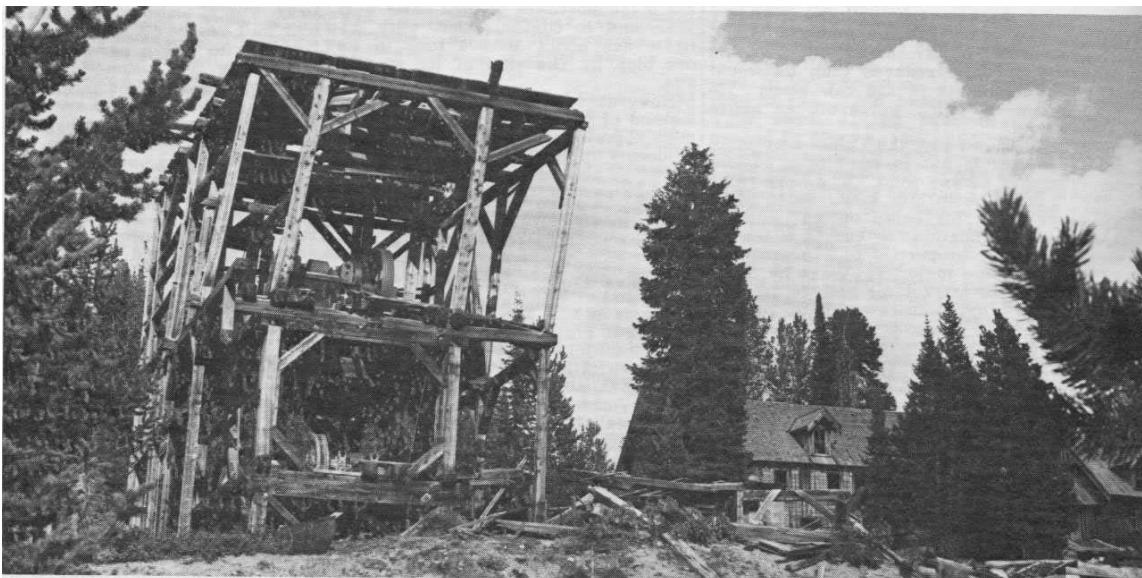
Figure 4-30. The lower tram's discharge terminal at the remains of the WS&P smelter, ca. 1960s (Glidden 1976).
