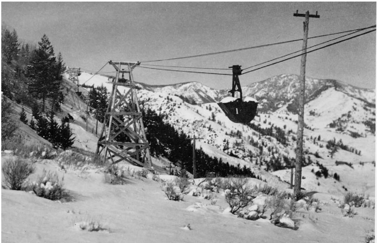
Figure 4-4. The Aldridge-to-Electric Bleichert Patent tram made by the Broderick and Bascom Rope Company. Photo ca. 1909 (Montana Historical Society Archives).
