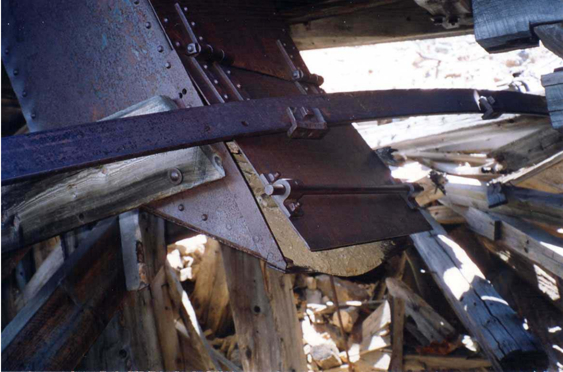
Figure 4-19. Detail of the ore metering device at the loading terminal.
