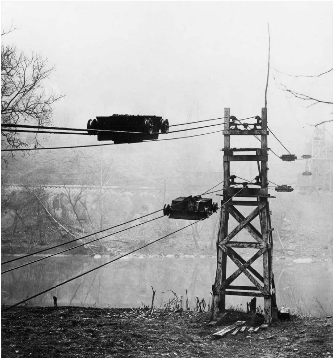
Figure 4-27. A Lawson style tram (Trennert 2001). The empty cars return upside-down on a lower set of parallel, static track cables. A small traction wire rope provides the drive.
