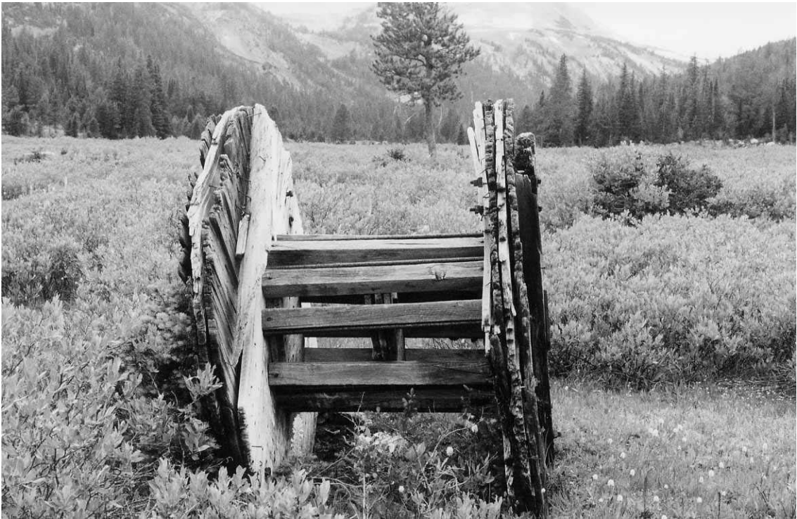
Figure 4-45. A cable spool lies along the tram route (1990 GCM file photo).
