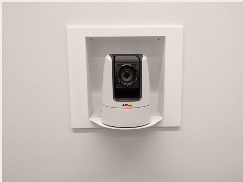
Break-Out Room Network Cameras (Pan, Tilt, Zoom)
