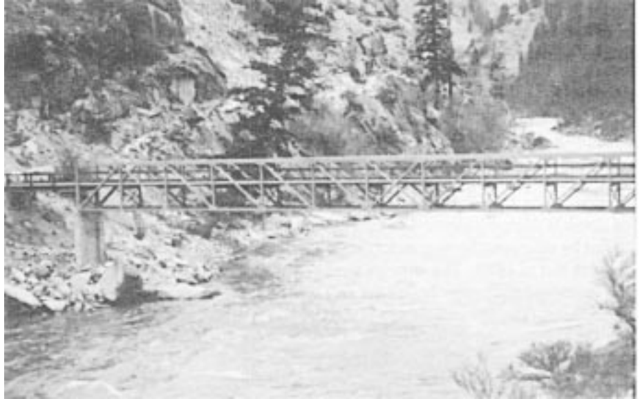
The Big Creek Bridge spans the Middle Fork of the Salmon River.
