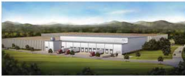
Winchester Cold Storage, Winchester, Virginia
