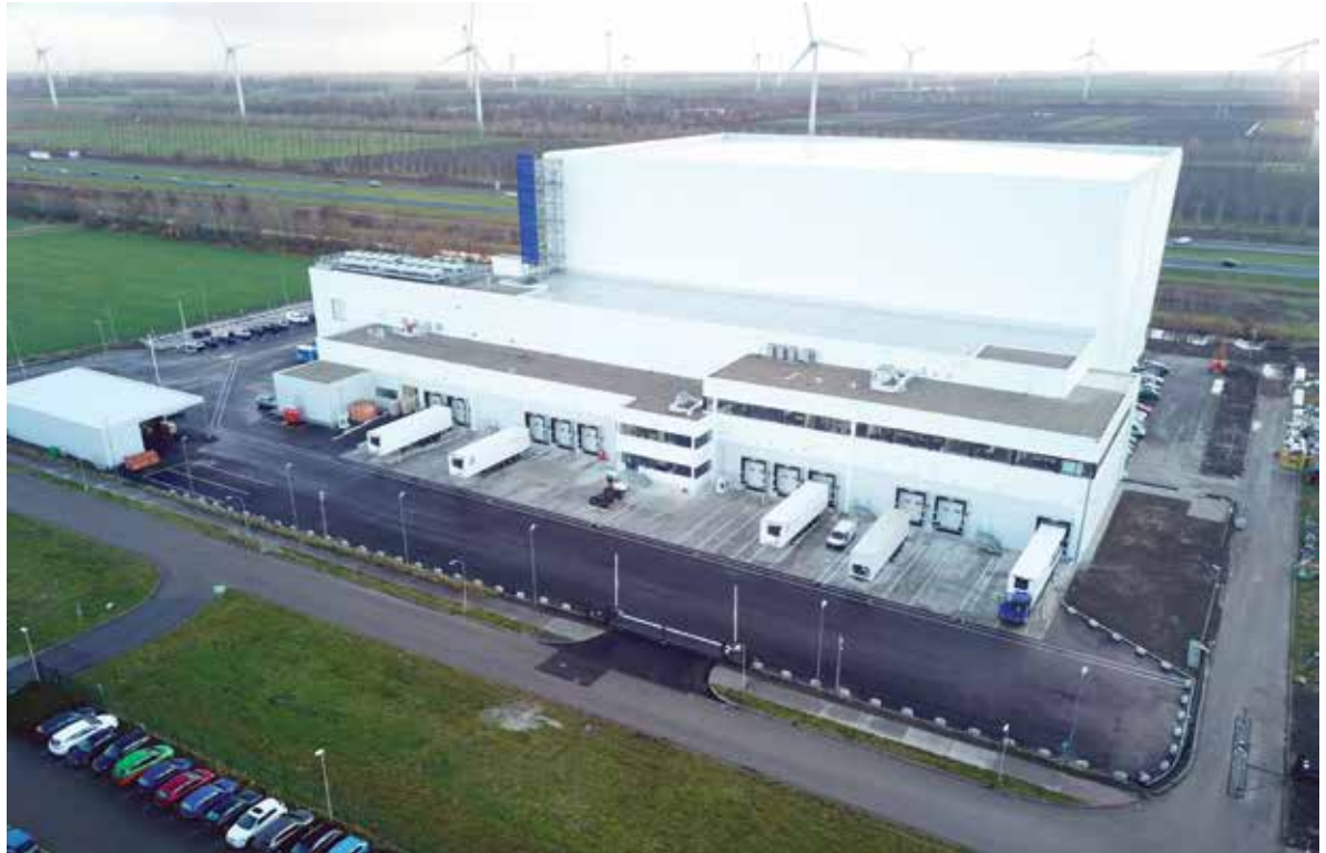
Left: Temperature-controlled warehouse with frozen and chilled chambers for pharmaceutical storage in San Paulo, Brazil. (Photo courtesy of Civil-Frio.)
