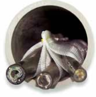
2" 3-Cell pack in 2" conduit
