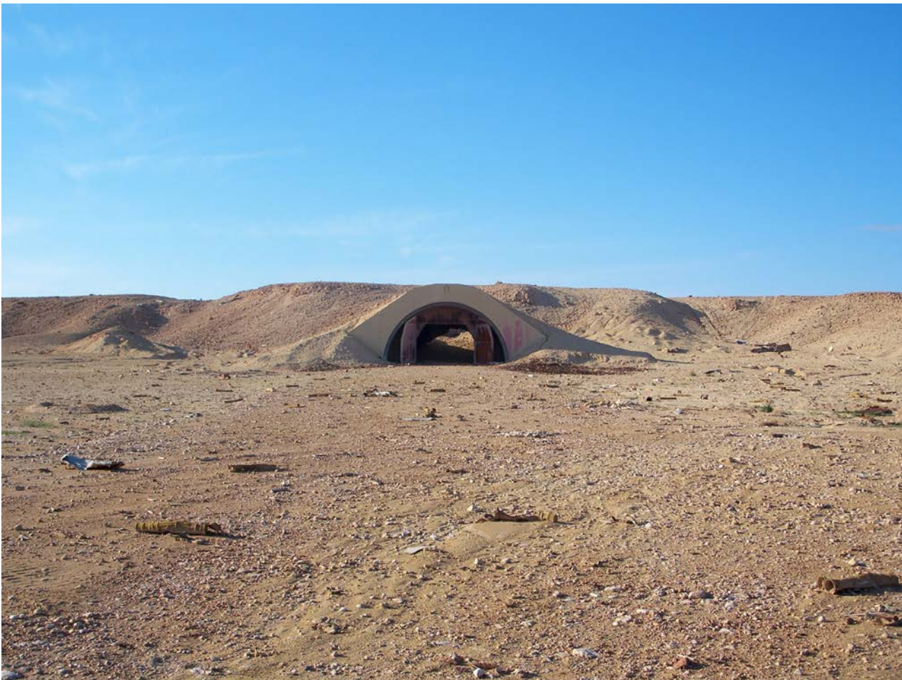
Figure 10.9 Arched steel magazine at Camp Wolf.
