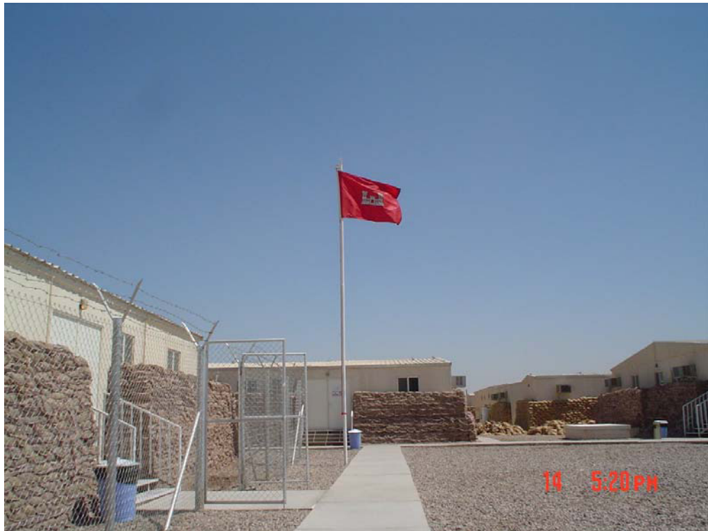
Figure 4.2 CEA/CMC headquarters at Camp Victory.
