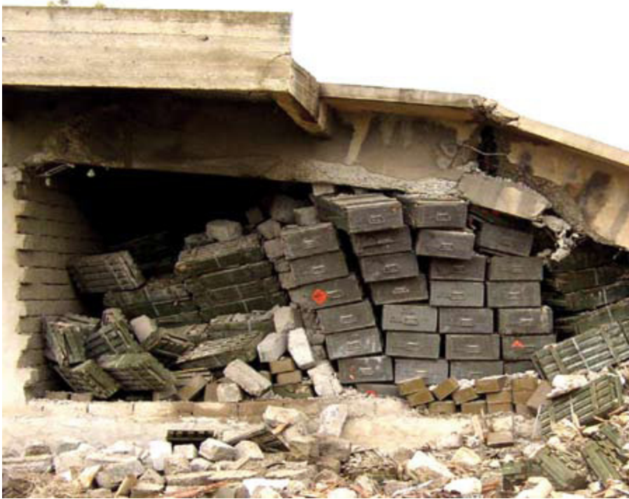
Figure 3.1 Remains of a munitions storage site.
