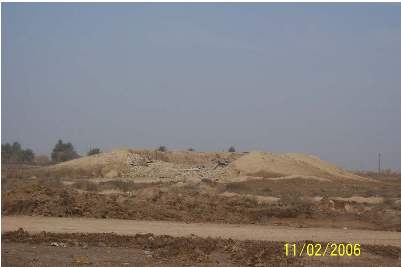
Figure 10.6 Collapsed ammunition storage bunker.
