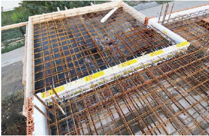
Thermally broken balcony
