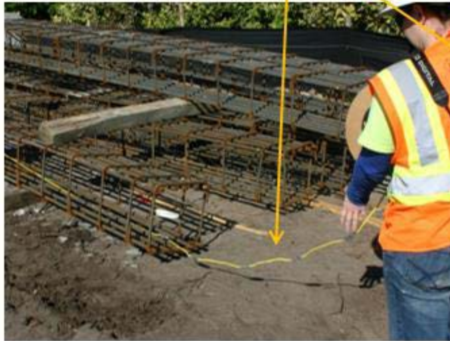
Method B - Uses Embedded wires attached to reinforcement cage
