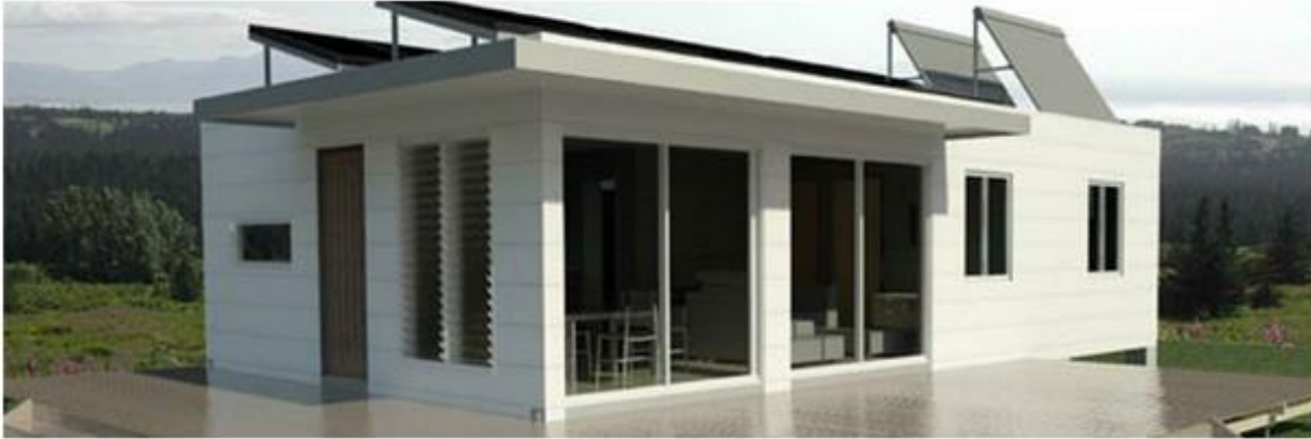
Figure 12 - Complete Modular Homes Granny Flat
