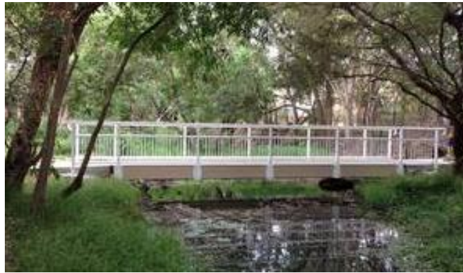
Figure 11 - BAC FRP Pedestrian Bridge
