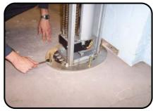
Using a hacksaw carefully cut the projecting bolt flush with the nut, ensuring the base plate is not damaged or marked in any way.
