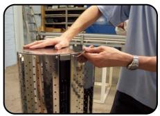
Before installing the Designer unit obtain four suitable fixing bolts, taking into account floor type and unit weight (see table 1)\*. Rawlplug <sup>®</sup> M10 Projecting Rawlbolt <sup>®</sup> 44356 type may be suitable. For dimensional details refer to the general assembly drawing, Figure 2.
