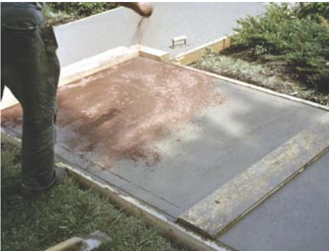
Dry-shake coloring compound is broadcast onto the surface by hand.
