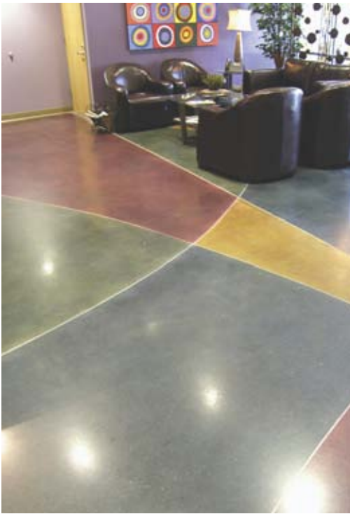
Preparation methods such as blasting with water or abrasives play a major role in the success of coating application to concrete surfaces. Photo courtesy of Dayton Superior Corp.
