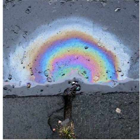
Photograph from Wikimedia Commons: Diesel spill on a road. Taken by Guinnog
