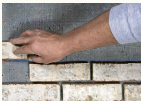
Adhesive interior installation on wood/steel stud backing.
