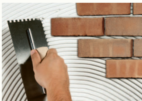
Interior or exterior mortar application on masonry or concrete.
