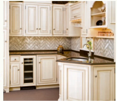
A Thin Brick backsplash in a herringbone pattern easily and dramatically enhances a kitchen.
