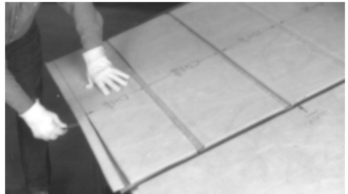
11. Using straight knife, cut through insulation and facing along last line - the line representing outer edge of closure flap. Peel insulation from flap. The board is now ready for assembly and closure to form a straight duct module or fitting.
