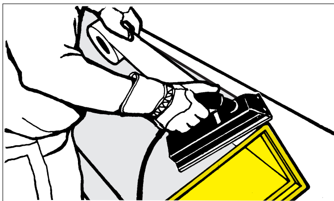
Fig. 5-4A. Apply heat with iron. Do not use a blowtorch; both heat and pressure are required for an effective bond. Complete the bond with a second pass of the iron.
