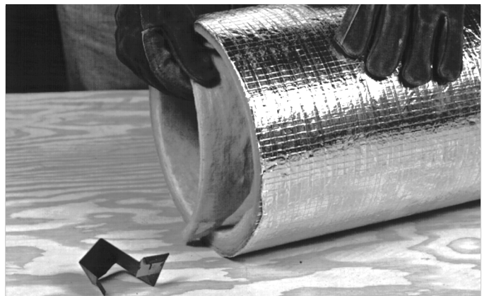
3. Using shiplap cutter to make female shiplap. Cutter is positioned to cut into inside of duct wall.
