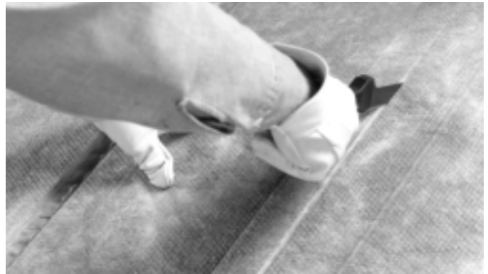
9. Using a straight knife, cut through insulation and facing along right hand cut. Peel insulation from closure flap. Board is now ready for assembly and closure to form a straight duct module.
