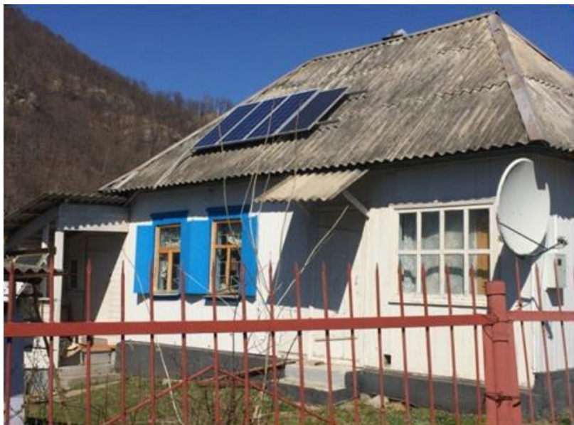
Figure 30 Autonomous rooftop PV system in Nikitino, an off-grid village in mountainous areas of Krasnodar Krai
