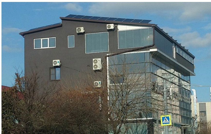
Figure 27 Hybrid PV-grid system; rooftop 30 kW PV solution on the roof of "Aloe Spa" Center in Krasnodar
