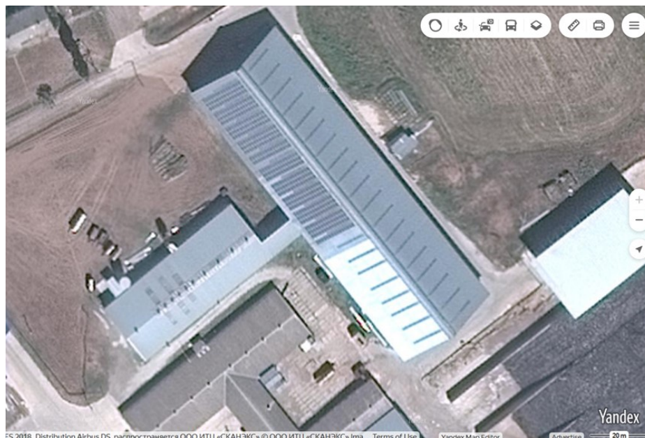
Figure 28 Satellite shot of a 100-kWp rooftop PV system in village Staronizhnestebliyevskaya in the middle of construction activities, 2019
