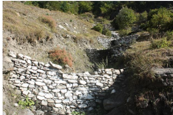
Photo 22: Loose stone check dam, Kaghan
