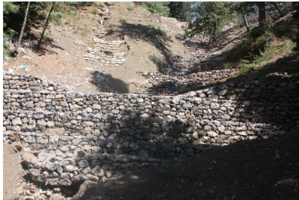
Photo 21: Gabion Check Dam, Gallies
