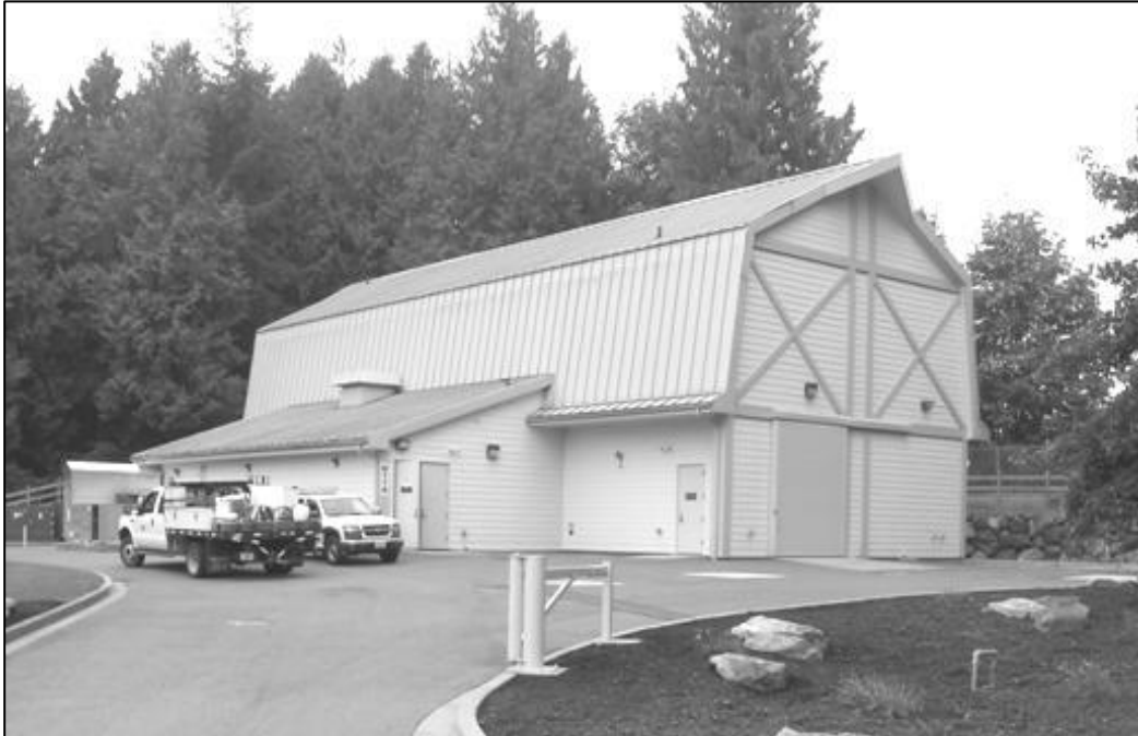
Clearview Pump Station from 64th Street SE, 2013
