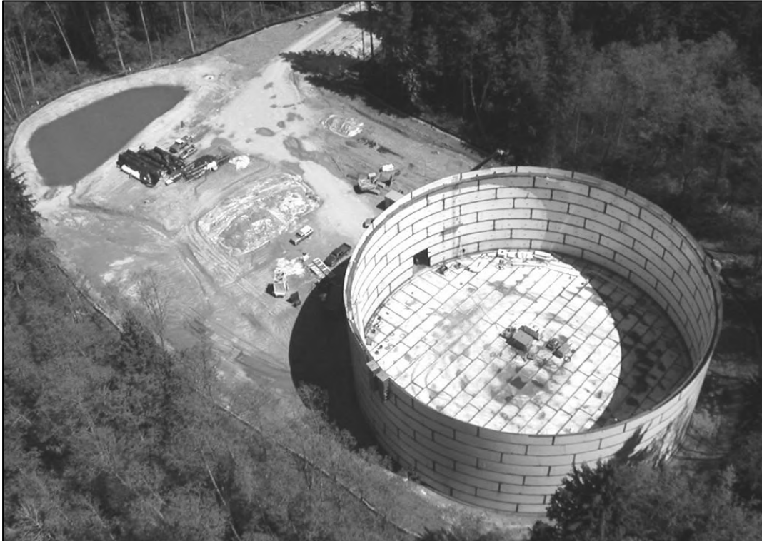
Clearview Reservoir During Construction, circa 2004
