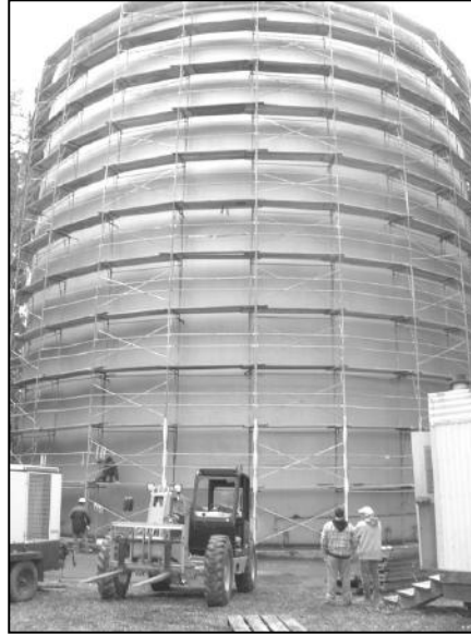
Canyon Park Tank During Recoating, 2005
