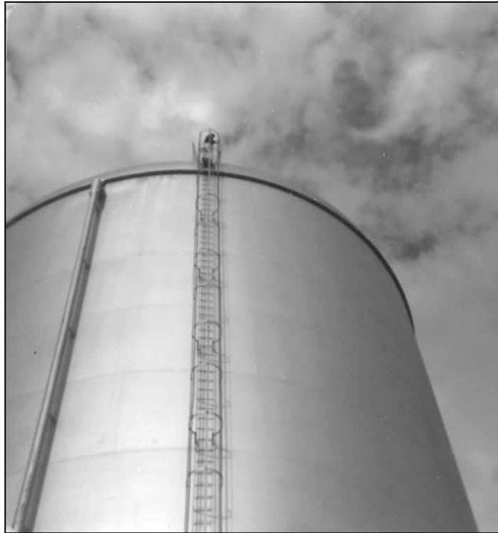
High Tank No. 1 with Safety Ladder, circa 1965
