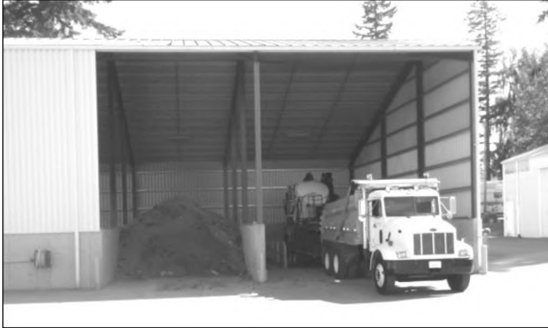
Decant Facility in Use, 2014
