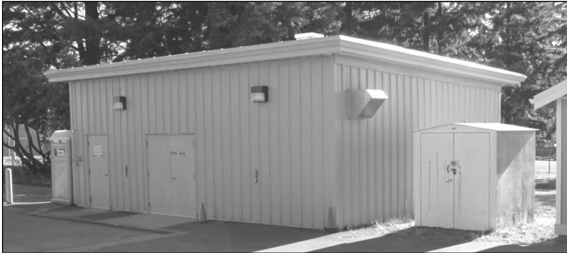
724 Booster Pump Station, 2014
