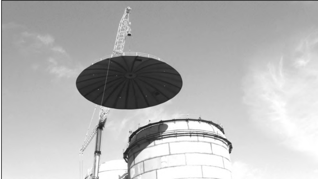
Crane Hoisting the Roof onto High Tank No. 2, circa 2002
