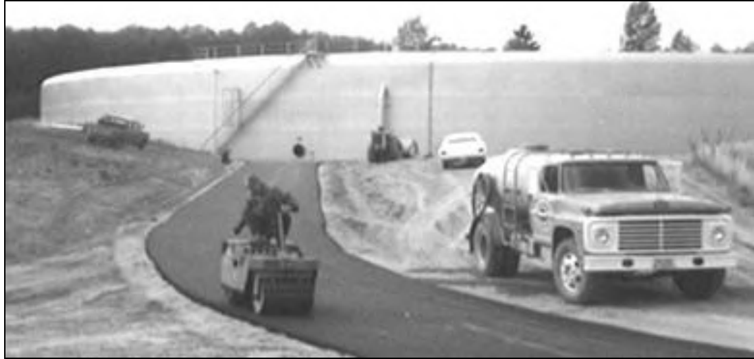
Paving the Driveway to Reservoir 3, circa 1977
