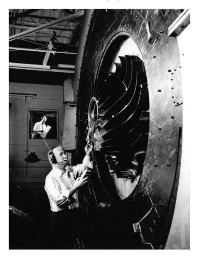
Figure 4-10. The Low-Speed Centrifugal Compressor Facility at Lewis. (NASA)
