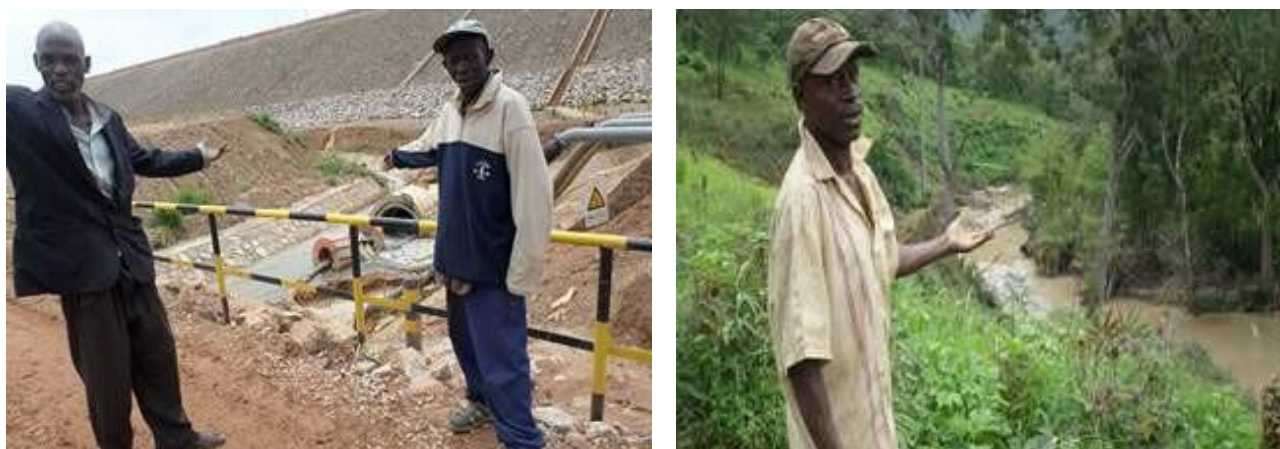
On the left, two inhabitants of the village of Yenge showing a canal and pipeline through which Sicomines' waste are poured into the Luilu river. On the right, an inhabitant of the village of Sept deplors the quality of the Luilu river waters at downstream.
