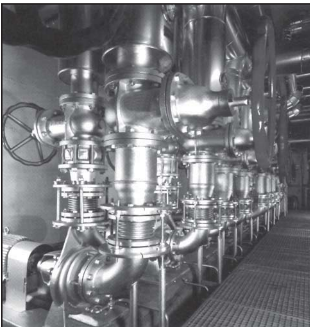
Typical pump station with a single bellows expansion joint system with control rods.
