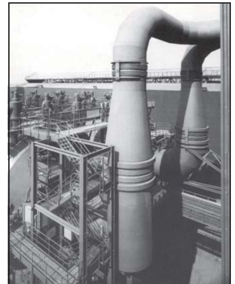
Thorburn's Hing-Flex expansion joints are designed for absorption of thermal expansion and wind loads.
