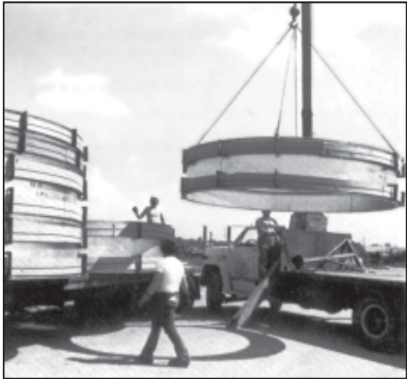
16' round environmental ducting expansion joints being shipped to an iron ore smelter application. Shown with protective covers.
