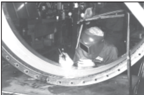
One of Thorburn's certified ASME Section IX welders in action
