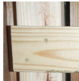
Figure 15 Diagonal Screw Placement
