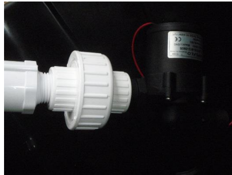
Figure 34- Class B Pump with Threaded Union
