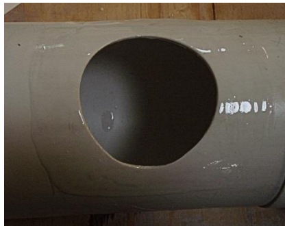
Figure 24 - Put Glue on Pipe
