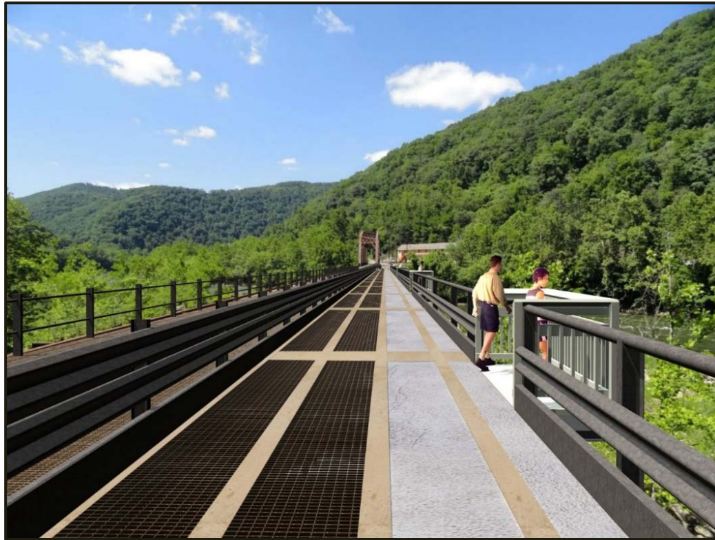
Figure 3. Selected Alternative (Renovation Alternative 4). This figure shows a computer generated depiction of the proposed renovation, including pedestrian refuge bays and concrete-filled strip of the roadway (by Michael Baker International for WVDOH).
