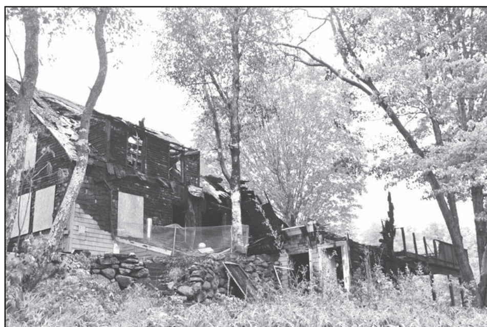
Fire destroyed a farmhouse on Peaked Hill Road in Bristol last Sunday afternoon, leaving little more than charred timbers remains behind.
