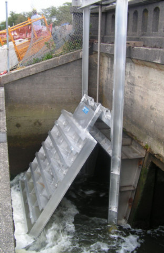
Photo 5 - Combination Gates were installed to replace existing timber flap gates on Highway 101 Bridge crossing the Chinook River.
