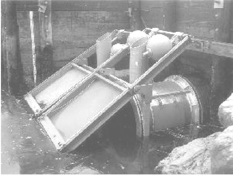
Photo 2- Self Regulating Tide Gate by Waterman Industries
